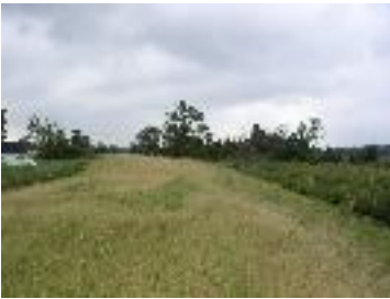
An earthen dike that was created in an earlier phase of the project.
